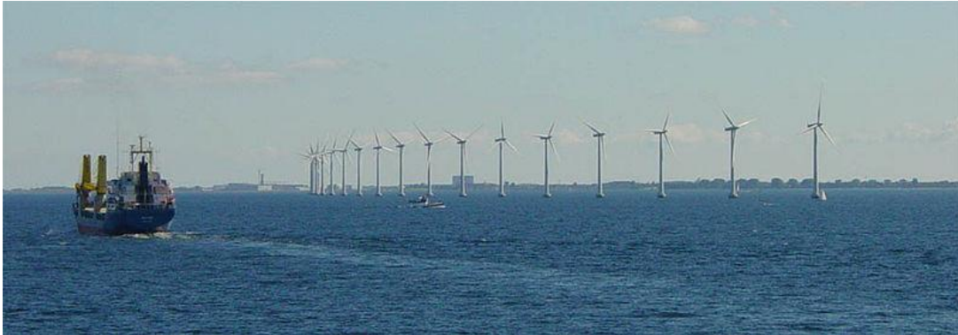
Figure 1. 6 An offshore Windfarm installed in Copenhagen(Denmark)
