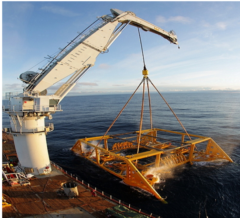
Figure 2.8: Subsea template in splash zone being filled (Statoil ASA 2012)
