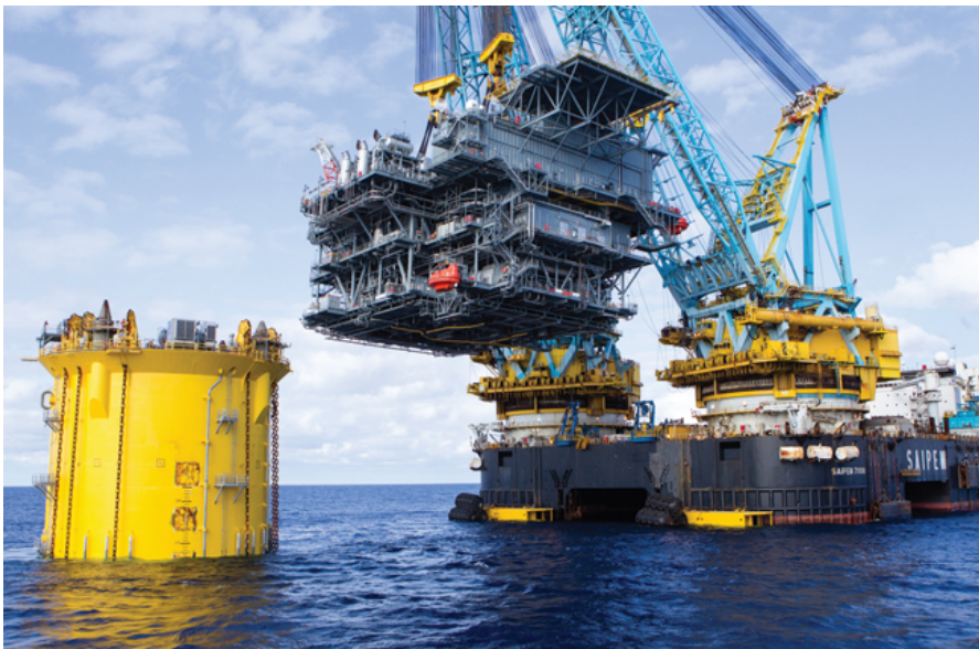
Figure 2.2: Lift of topside Saipem 7000 (Boyd 2015)
