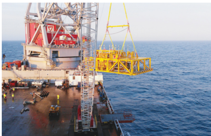
Figure 2.7: Subsea compressor moved into lowering position (Statoil ASA 2015)
