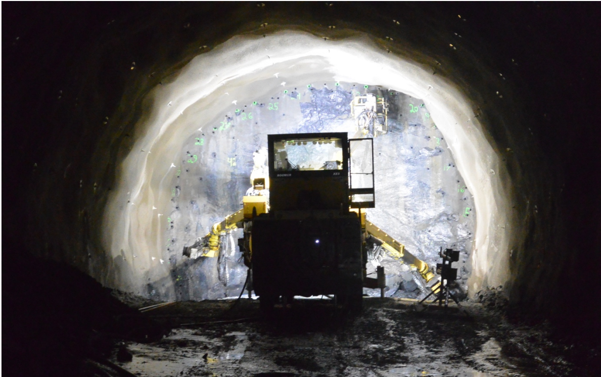
Figure 1.1 Drill and blast method - drilling jumbo at the face
