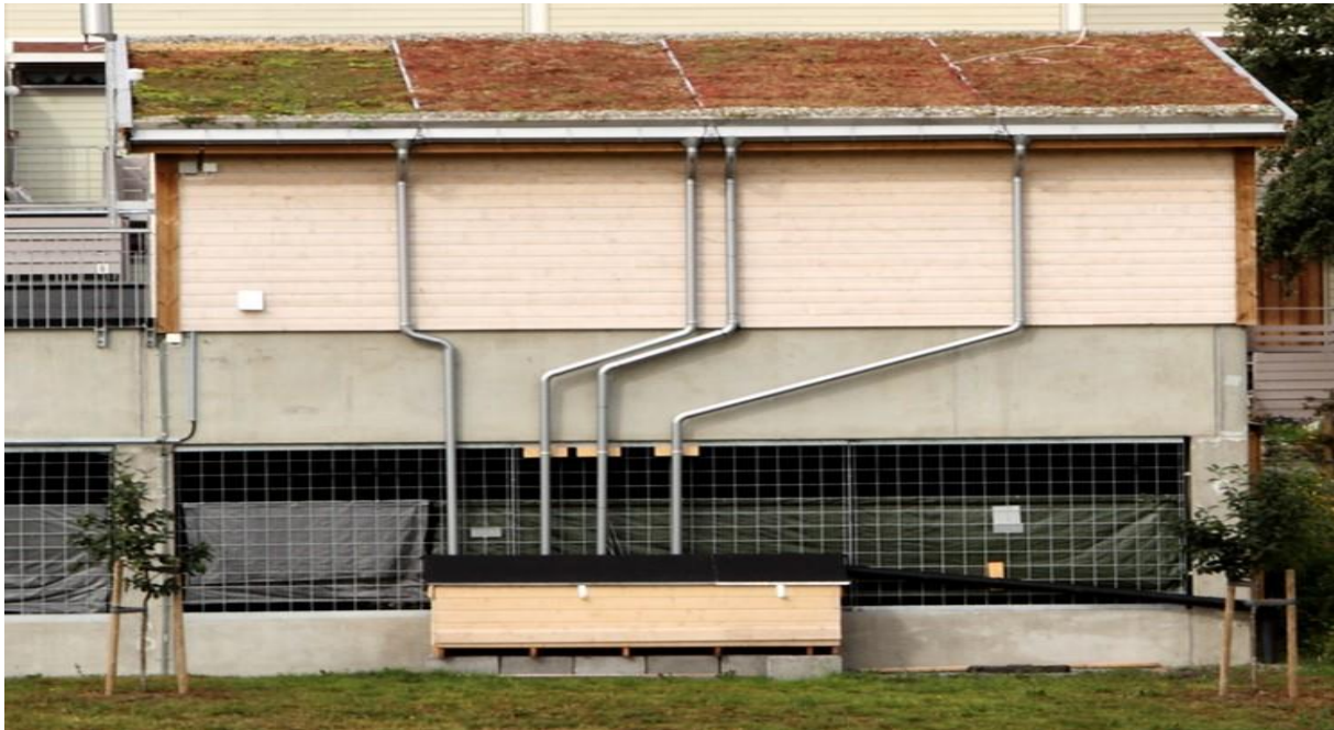
FIGURE 1.1 THE GREEN ROOF SITE AT RISVOLLAN, TRONDHEIM. THE ROOF IS DIVIDED INTO FOUR PLOTS, WITH THE PLOT AT THE LEFT BEING NAMED 'PLOT 1', AND FOLLOWING FROM LEFT TO RIGHT WE HAVE 'PLOT 2', 'PLOT 3' AND 'PLOT 4' (IVM, 2014).
