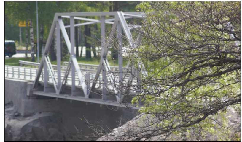
Bridge threatened by September, 2015 flood near Omnessfoss
