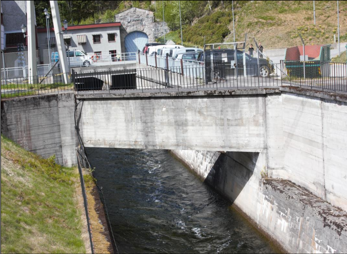
Tail water from Mar Hydropower Plant
