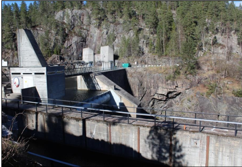
Spillway of Vrangfoss
