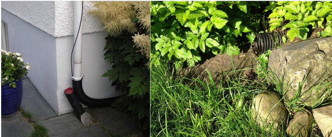
Figure 3.2 Downspout disconnection. The picture to the left shows how the downspout can be disconnected from the sewer system. The water is then led through a pipe to an appropriate infiltration surface were the water can infiltrate, like shown in the picture to the right. (Photo: Bent C. Braskerud)
