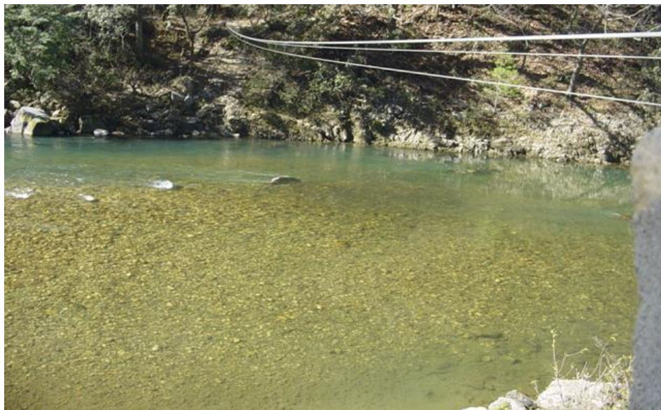
Picture 4.1: Cableway facilities installed at Tamchu sediment gauging station at Tamchu (Source: DHMS, MoEA, 2015)
