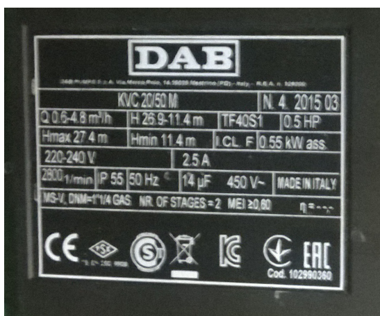
Figure 4.7: Characteristics of the pump DAB KVC 20/50 M
