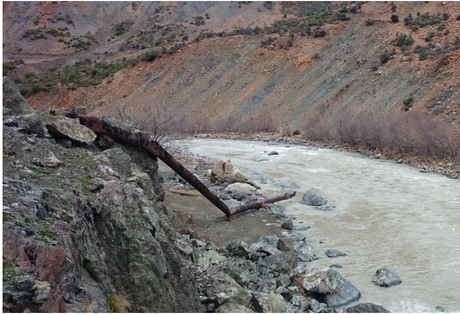
Figure 2.5 Former siphon pipeline from Bratile Reservoir. Photo: Christian Almestad
