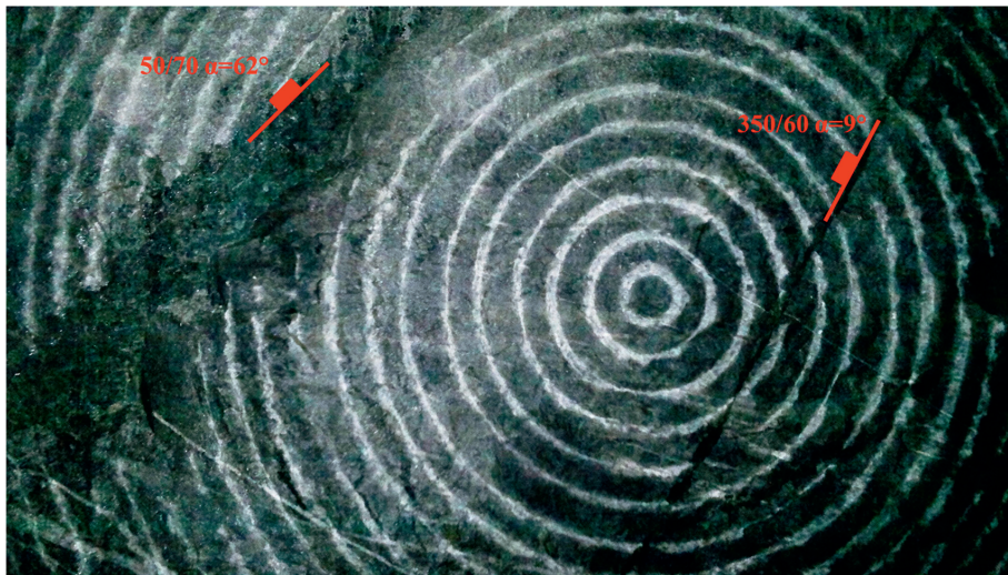
Figure 75. A photograph taken during a tunnel face inspection showing void areas generated after tunnelling in a fractured rock mass. The tunnel axis orientation is 160 degrees. (Photo courtesy of Tobias Andersson).
