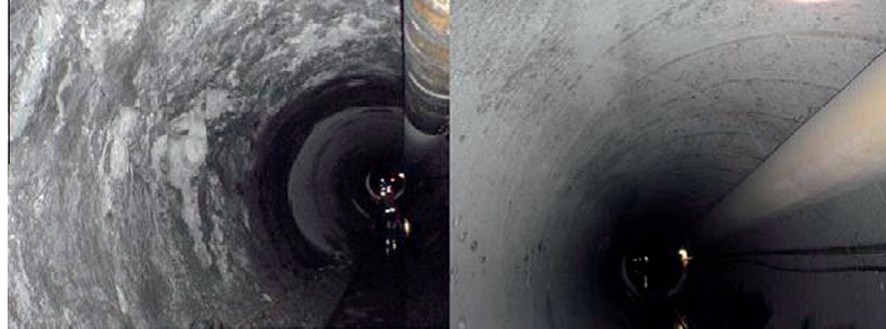
Fig. 13. Examples of high (left) and low (right) k_s tunnel values.
