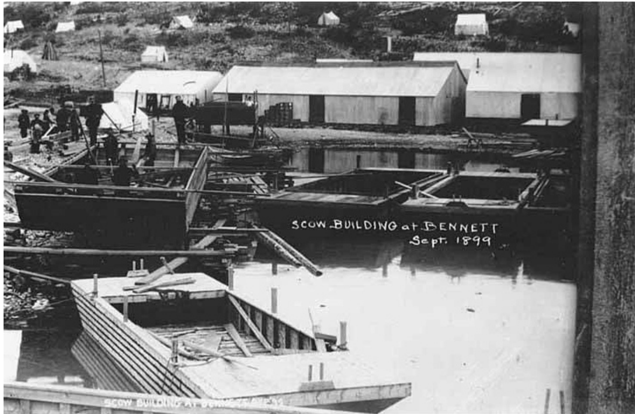
Figure 17. Klondikers constructing scows at Bennett, British Columbia, September 1899. (University of Washington Libraries, Special Collections, AWC1707)
