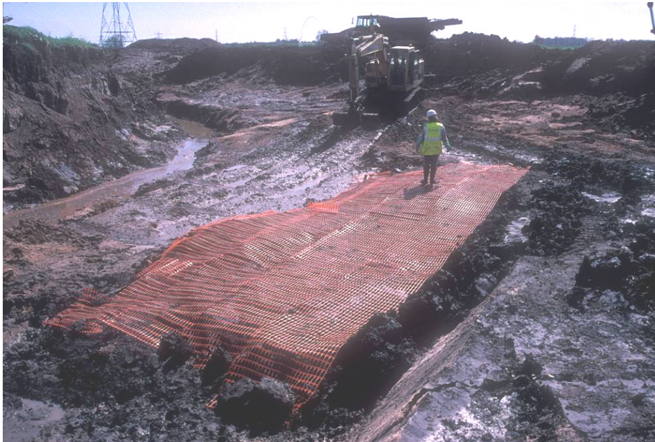
Figur 12: The netlon ® demarcation layer placed over the silt mound over the second Shardlow Boat. Photo: Birmingham Archaeology (Williams 2008:321).
