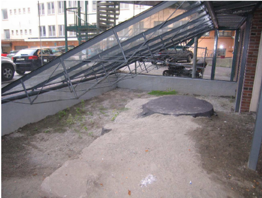
Figure 11: The western part of the Katarina Hospital in Bergen covered with geotextile and sand. The glass roof now protects the remains from rain. Hommedal is of the opinion that the ruins should be uncovered and displayed like the rest of the ruins (Hommedal 2007:11).
