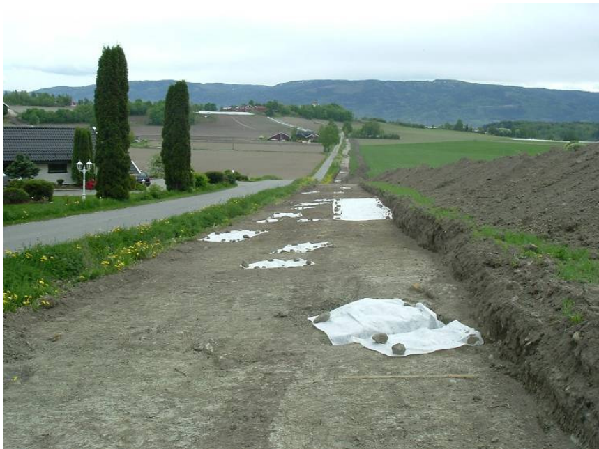
Figure 1: Cooking pits revealed during topsoil stripping covered with geotextile. Photo: Buskerud County Municipality. Date 14.05.2008.
