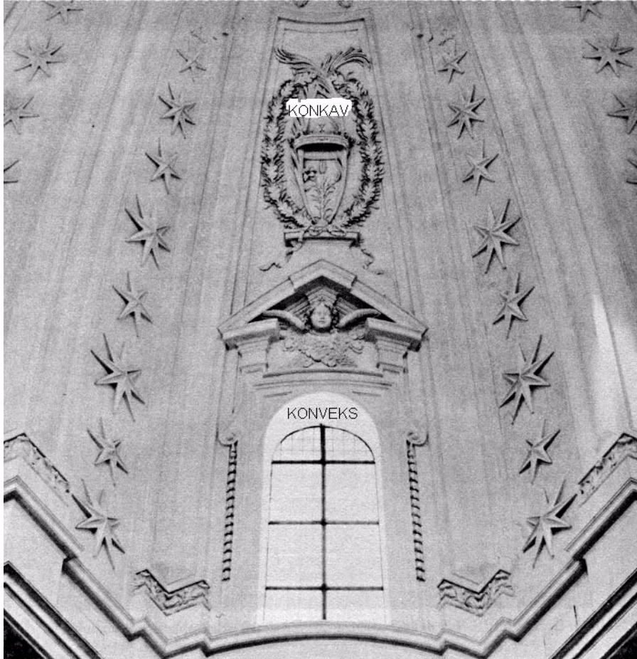
Fig. 2. Sant'Ivo, interior; transition from main body up to the cupola, from convex to concave (in Norwegian but hardly difficult).
