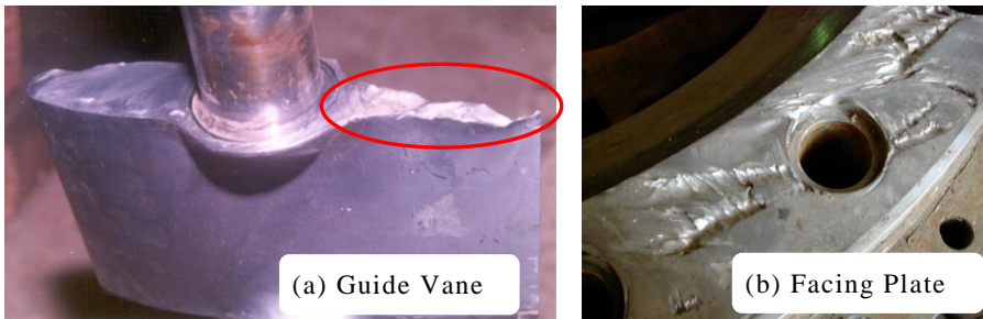
Figure 1. Erosion of GV and facing plate in Francis turbine [18]
