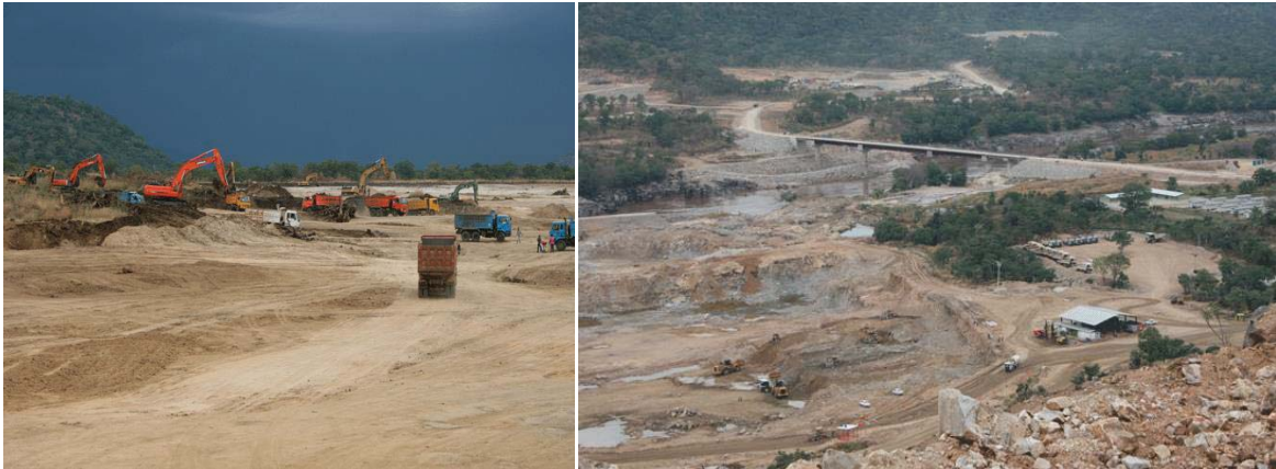
Figure 4.1 Soil exposure due to construction activities
