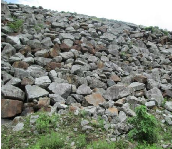
Figure 6.15 Existing rock fill of prototype Kulekhani of downstream slope
