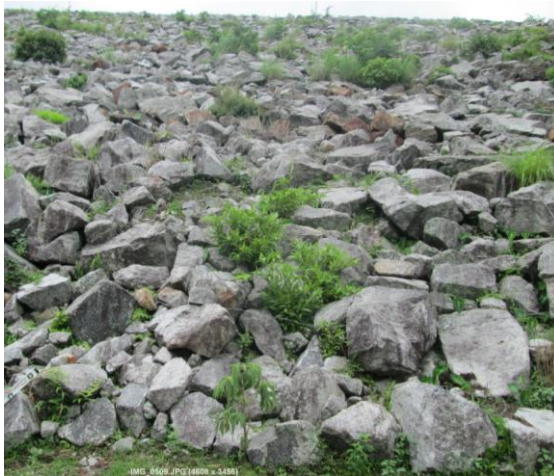
Figure 6.17 Existing rock fill of prototype Kulekhani of downstream slope
