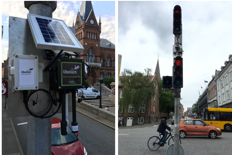
Figure 4: Sensor deployment on traffic lights in Vejle city center, showing full deployment on a mounting plate with platform, solar panel, and downward facing sensors for \text{CO}_2 ; \text{NO}_x ; combined Temperature, Pressure, Humidity; and combined \text{PM}_1 , \text{PM}_{2.5} and \text{PM}_{10} (the separate box on the left)
