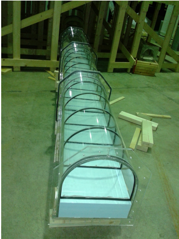
Figur 3.4: Tunneldelene under montering.
