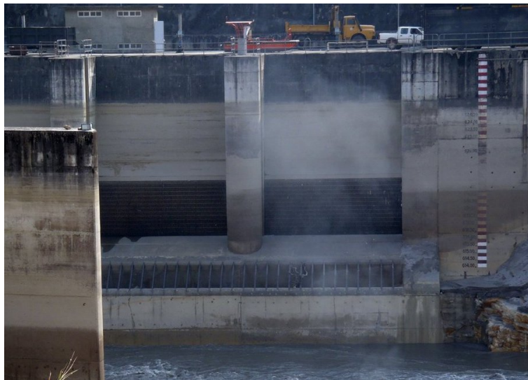
Figure 3.17: Bed control solution at Middle Marsyangdi
