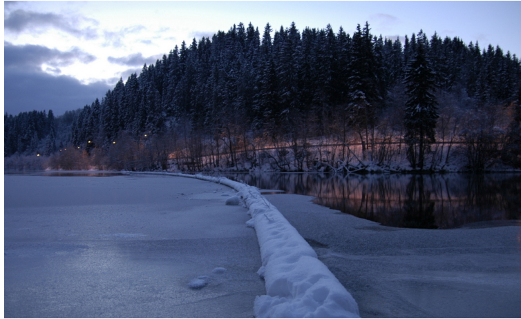
Figure 2.2: Floating boom at Nedre Leirfossen power
