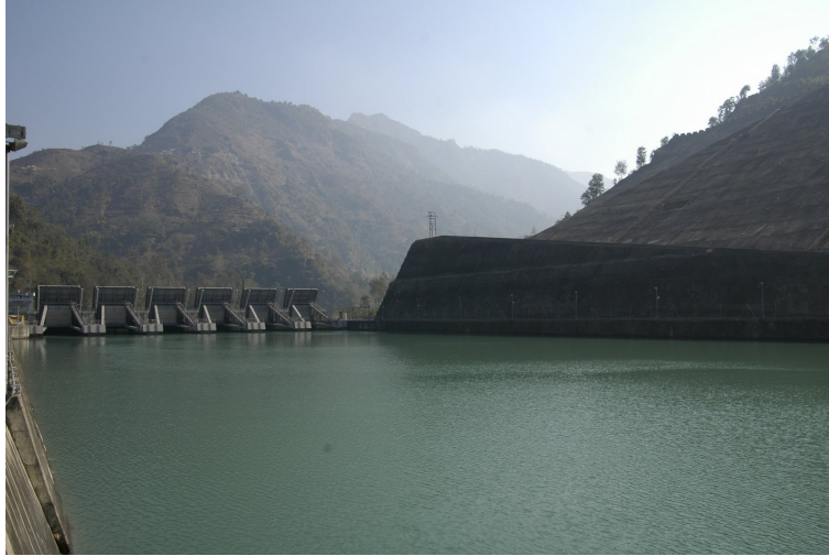
Figure 3.26: The settling basins at Kali Gandaki
