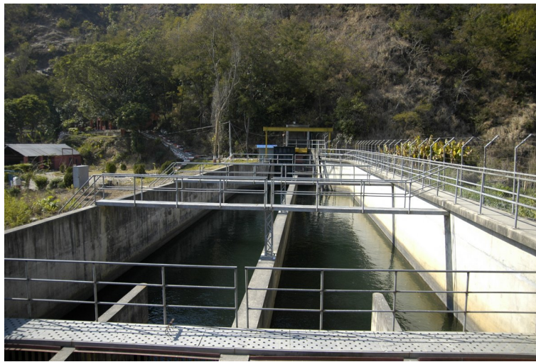
Figure 3.4: Settling basin at Jhimruk in Nepal
