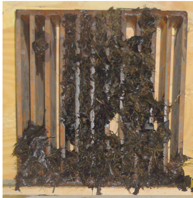
Figure 2.17: Trash rack after flushing test 1
