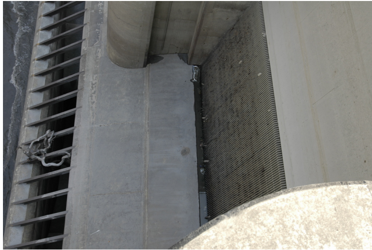
Figure 3.10: Undersluice slot at Middle Marsyangdi HEP
