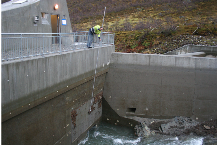
Figure 2.3: Manual raking of trash rack
