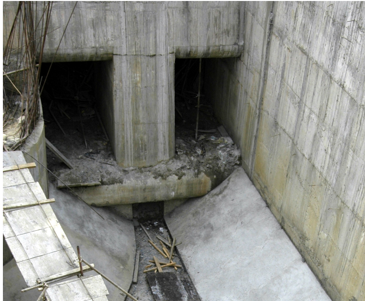
Figure 3.19: Flushing channel at Lower Modi HEP
