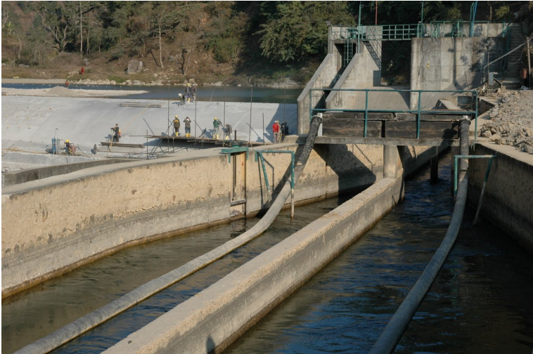
Figure 3.7: The Serpent Sediment Sluicing System at Andi Khola in Nepal
