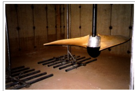
FIGURE 2.10 MBR AERATION SYSTEM WITH DIFFUSER AND MIXER. [30]
