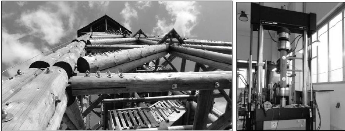
Figure 25: Watchtower near Lázně Bohdaneč (left), setup round timber bolted joint with slotted-in plate (right)
