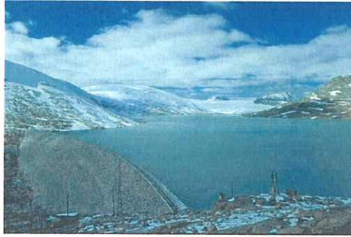
Figure 2.6 A typical Norwegian rockfill dam, Styggevatn Dam, with Jostedal Glacier in the background (photo: Statkraft)
