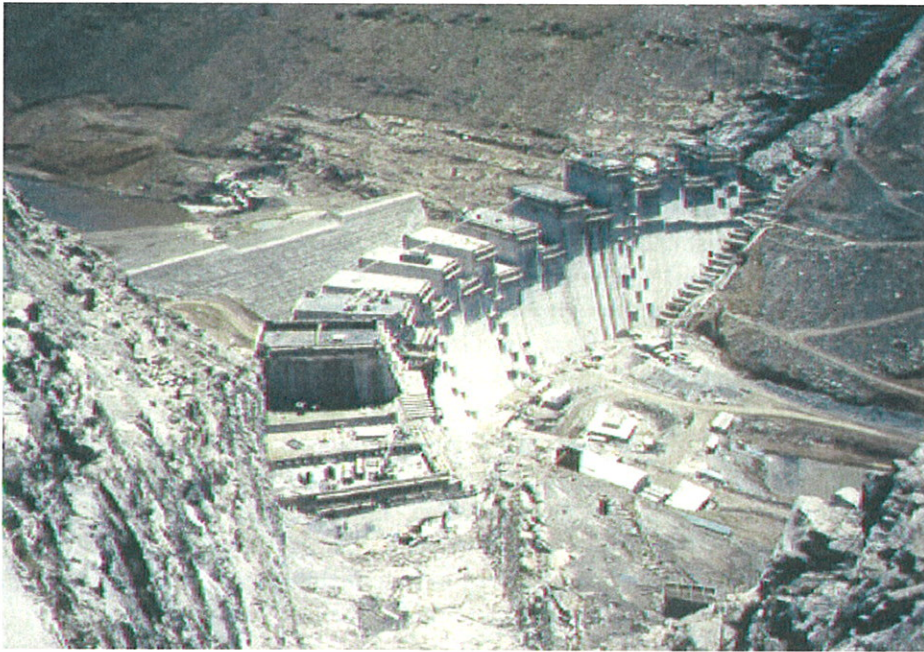
Figure 1.1 Construction of Katse Dam, Lesotho, November 1994
