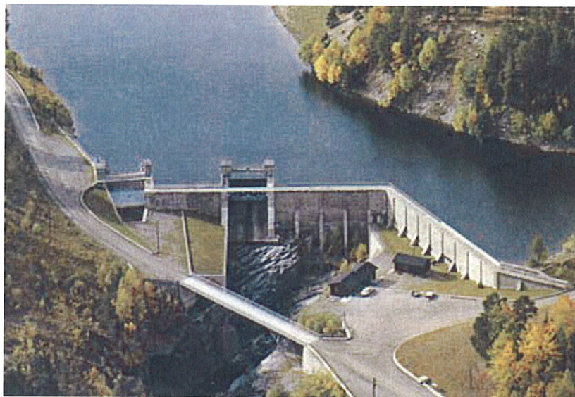
Figure D-7 Olstappen Dam (photo: GLB)
