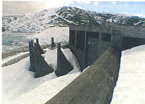
Figure 2.8 Styggevatn Dam and spillway, 24 June 2001 (photo: H.M. Kjellesvig)
