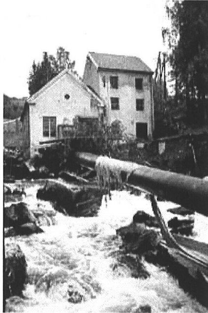
Figure B-5 Moksa 1 and the pipeline, where the river broke through the river bank
