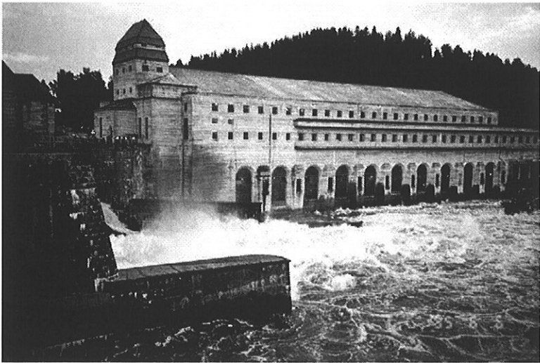
Figure B-13 Solbergfoss Dam and power plant (photo: P.C.Røhr)
