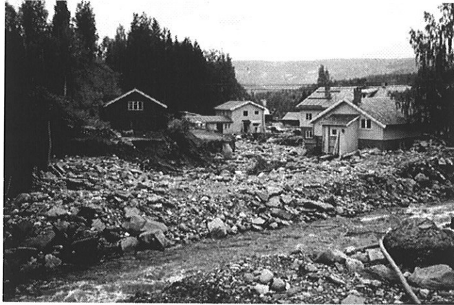
Figure B-3 Damages caused by the flood – downstream reach of the new river course
