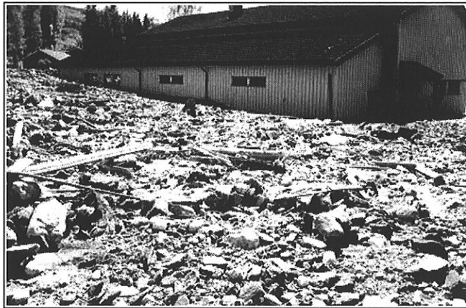
Figure B-2 Deposits upstream of Moksa power plant after the flood (photo: MGE)
