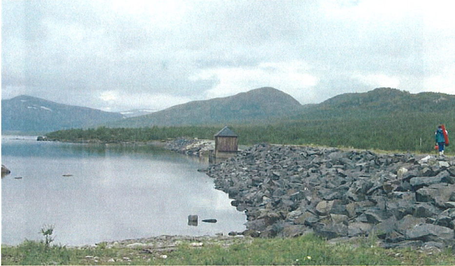
Figure D-5 Øyvassoset Dam and part of the Kaldfjorden Reservoir
