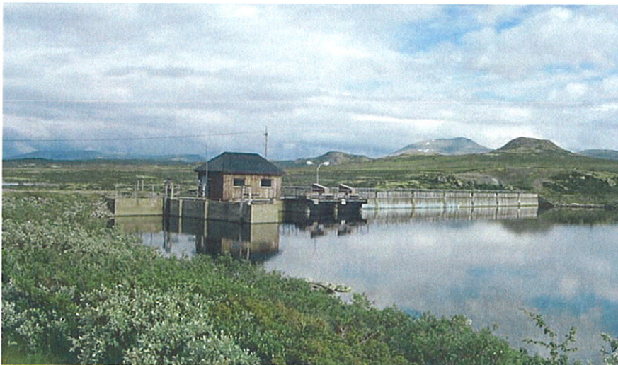
Figure D-4 Vinsteren Dam seen from the upstream side
