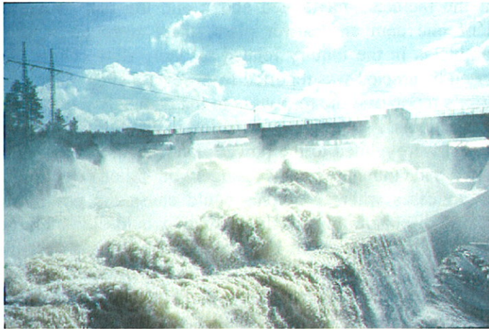
Figure 5.15 Peak discharge at Vamma Dam during 1995 flood
