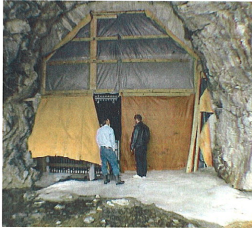
Figure 2.7 Insulation of spillway tunnel outlet at Styggevatn Dam (photo: H.M. Kjellesvig)
