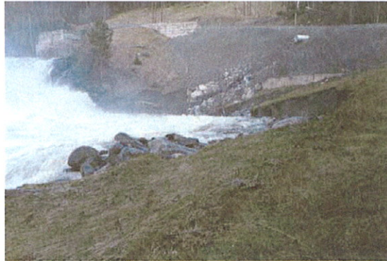
Figure D-9 The 1987 flood downstream of Olstappen (at Kamsfossen) – erosion of river bank (photo: O.P.Dahle, GLB)
