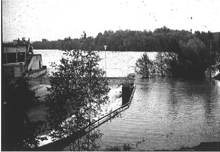
Figure B-12 Bingsfoss Dam and power plant, high upstream water level
