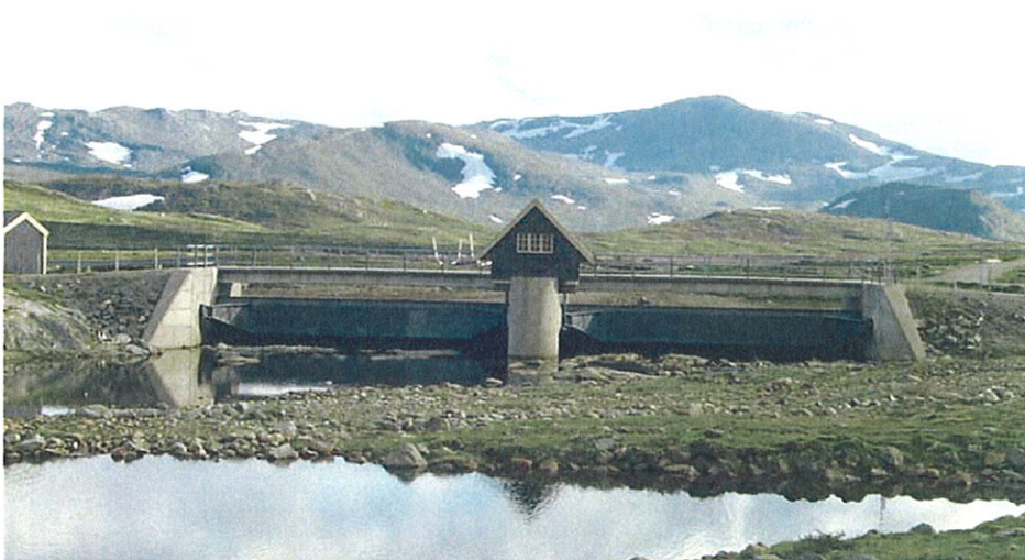
Figure D-2 Bygdin Dam with two radial gates
