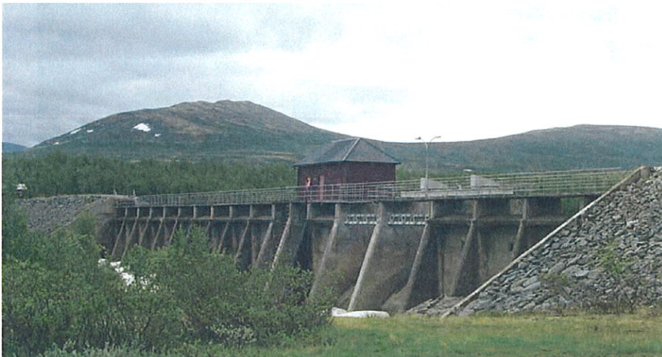
Figure D-6 The spillway section at Øyvassoset Dam
