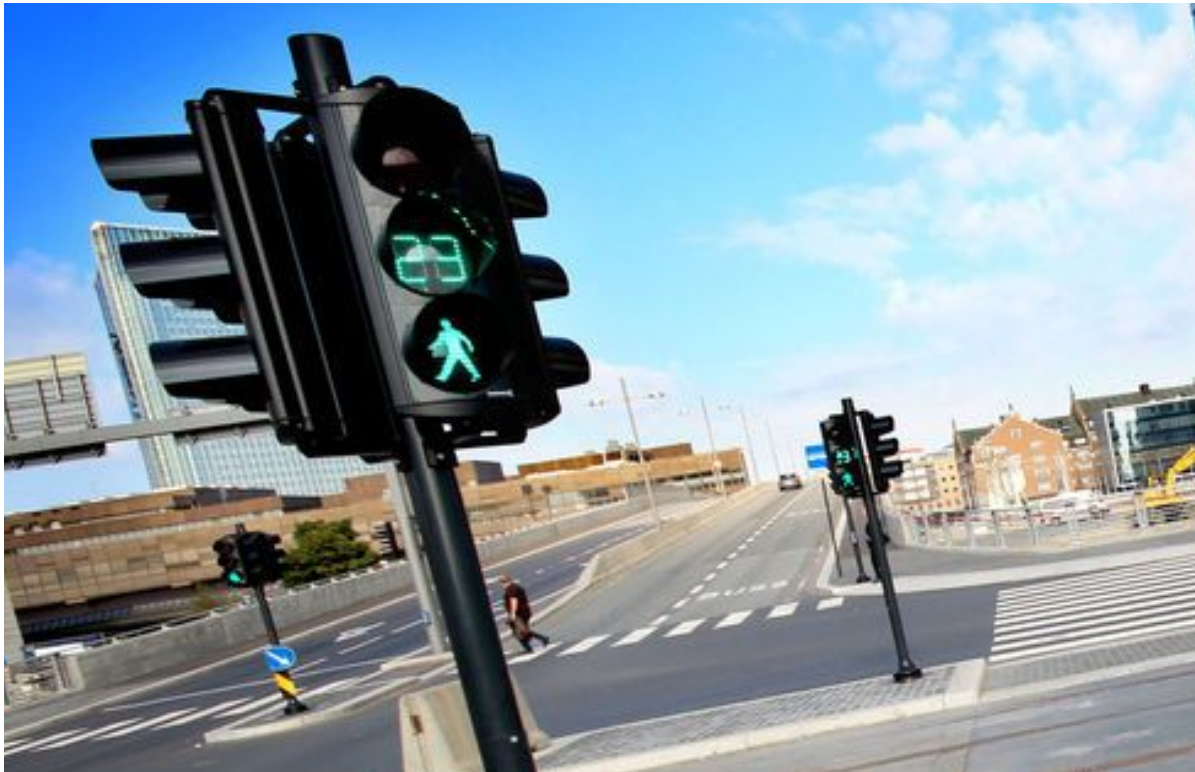
Figure 2.4: Automated crossing with countdown timer. Timer shows green light signaling the street is open for pedestrian crossing. (Source: http://www.dinside.no/930507/tester-gangfelt-med-nedtelling Image by: Ole Petter Baugerød Stokke. Image is subject to copyright and used per agreement).
