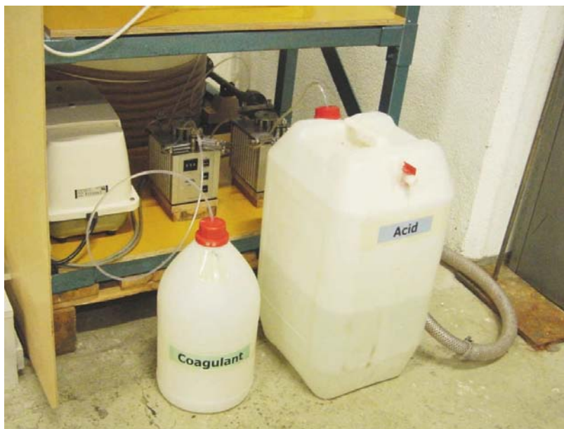
(b) Coagulant dosing station and air blower (left)
