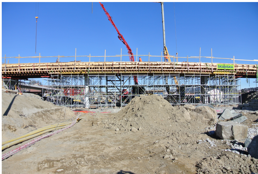
FIGURE 5.1: Photography of Sandsgård bridge right before casting of the edge beams.
