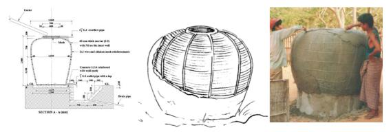
As with the ferro-cement tank there is the need for skilled labor, however the water pots are made smaller than the tanks and may be constructed elsewhere and transported. It is relatively cheap in materials and is relatively quick to construct.
