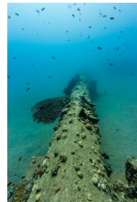
Figure 7.1: Pipeline example image. Courtesy of ( Subsea Pipeline Inspection, Repair and Maintenance - Theon - Oil and Gas Front End Consultancy & Petroleum Engineering Consultants — Theon - Oil and Gas Front End Consultancy & Petroleum Engineering Consultants , 2016).
