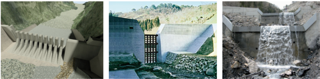
Figure 2.5: The left picture is a concrete slit dam in Madeira, Portugal (LCWConsult, 2015). The middle picture is a grid dam (Nippon steel and Sumikin metal production, 2016) and the right picture is a series of closed check dams (Remaître et al., 2008).
