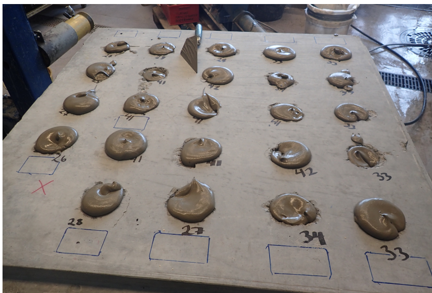
Figur 9.14: Hullfylling. Klart for å sette inn stag.
