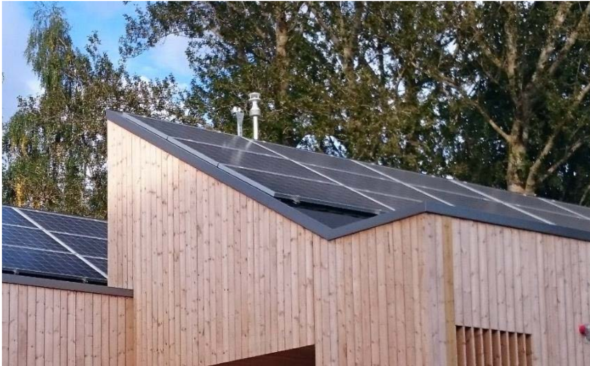
Fig. 1.14. Weather station installed on the south roof of the ZEB Living Lab (Good 2015).
