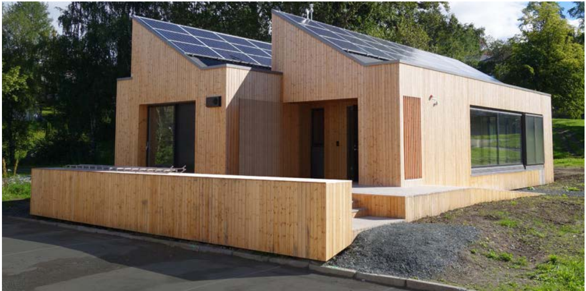
Fig. 1.9. The ZEB Living Lab at NTNU (Norwegian University of Science and Technology) in Trondheim (Finocchiaro et al. 2014).
