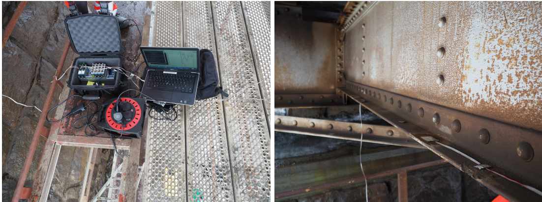
(a) System setup from data gathering at Lerelva (b) Placement of strain gauges on stringer section
