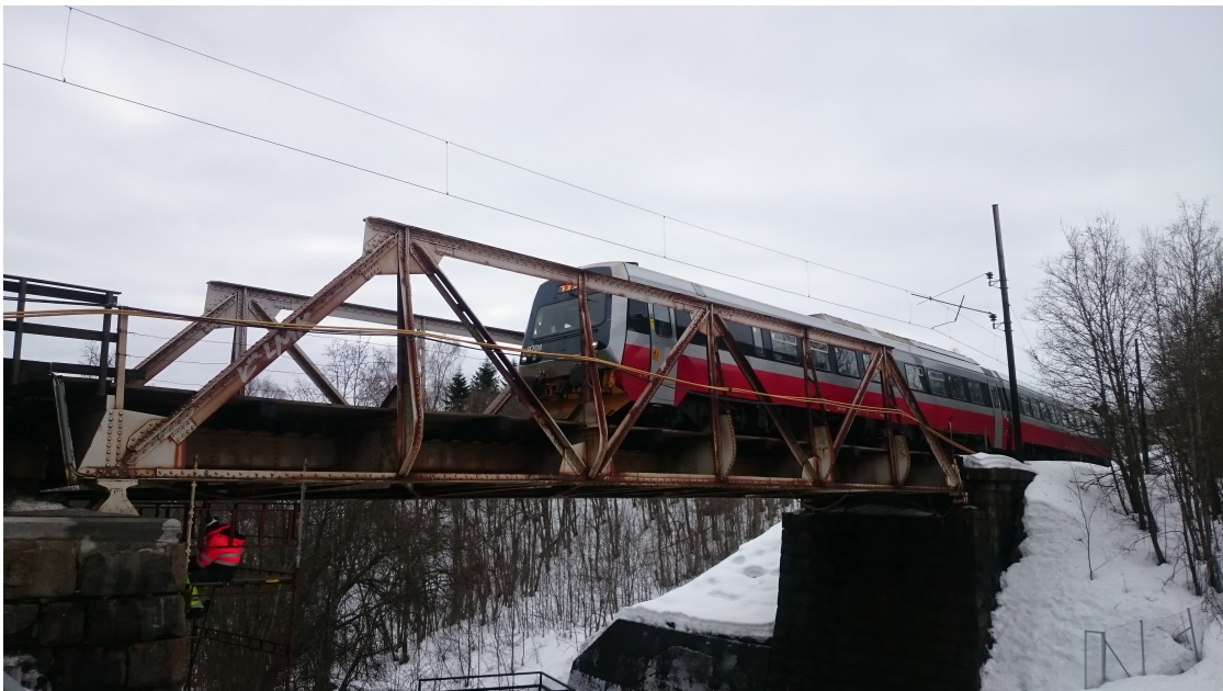
Figure 3.5: Lerelva bridge with a train passing over
