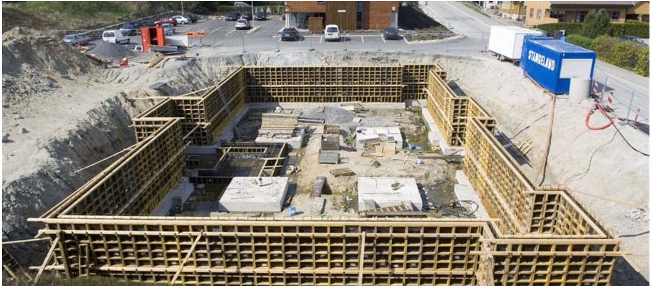
Figur 9 - Forskalingsform. (12)
