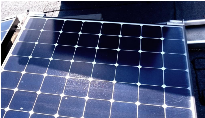
Figure 6.14: Cast shadow from the exhaust vent at Block 5, affecting string B5_V4B. Taken May 10th, 15:34 .
