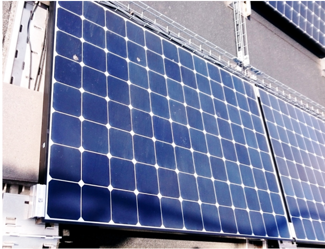
Figure 6.20: A photo showing the shading by the weather station. Taken May 10th, 16:07.
