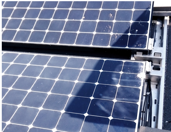
Figure 6.16: Cast shadow from the open roof hatch, affecting string B5_V1B and string B5_V3B. Taken May 10th, 10:24.
