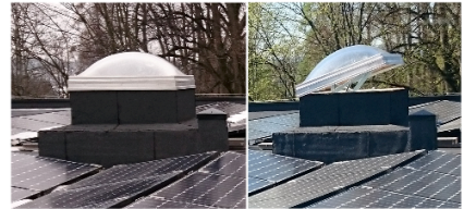
1. Roof hatch closed/open
