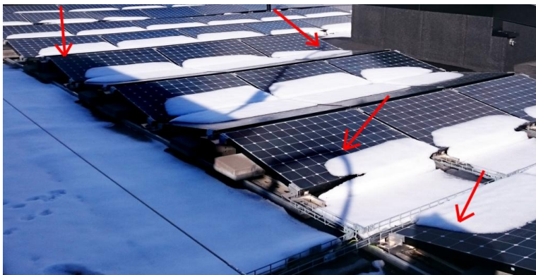
Figure 2.9: Cast shadow from the weather station and parts of the building, 13:15 March 8th. (Photo by L. Ødegården)
