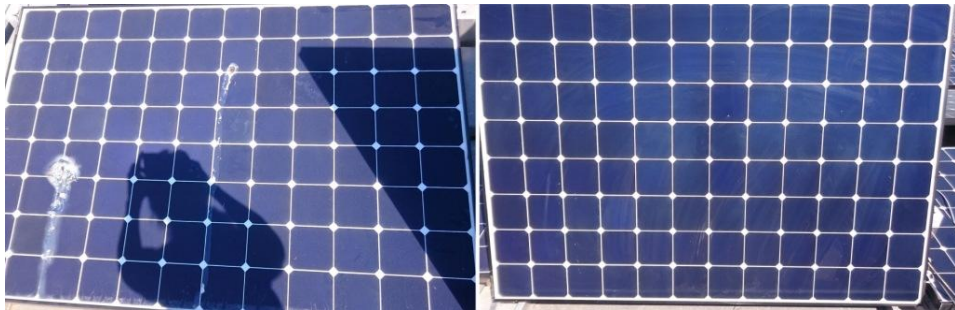
Figure 6.7: Photos showing the PV module before (left) and after (right) cleaning.
