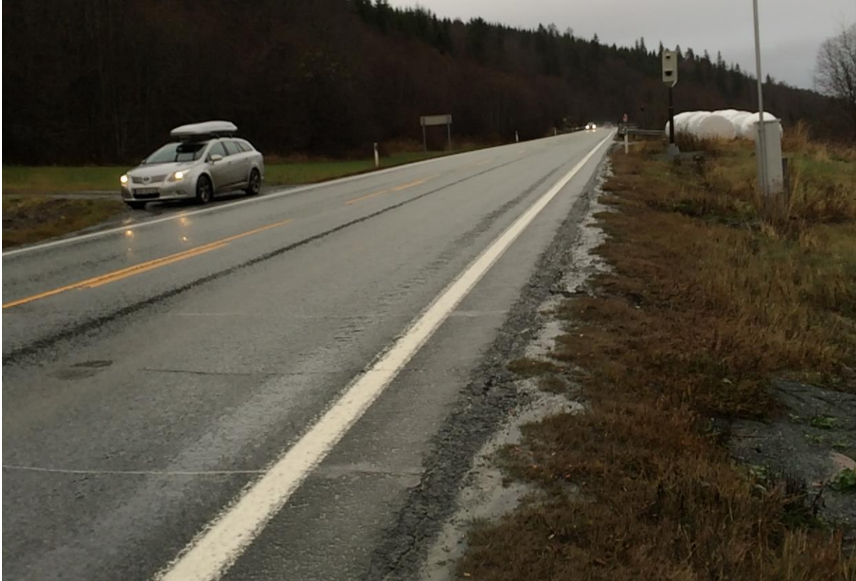
Figure 8: Picture of WIM 1740009. The two transversally laid WIM cables can be seen in the front of the picture. Photo: Torbjørn Haugen.
