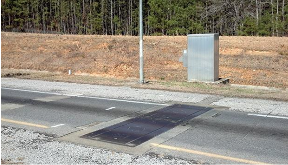
Figure 2: WIM bending plates scale. Figure: IRD. 27
