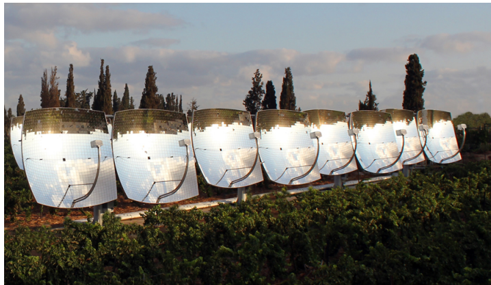
Figure 2.16: Zenith Solar collectors operating in Israel. The area of the collectors covers 22 \text{ m}^2 and the orientation follows the sun (From Zenith (2006) ).
