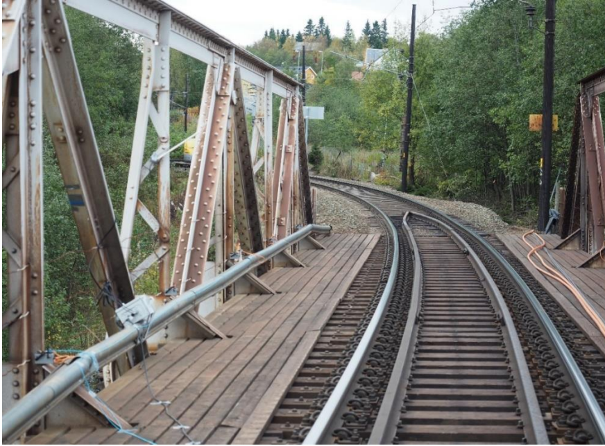
Figure 31, extra set of rails and inspection deck. Photo: Gunnstein
