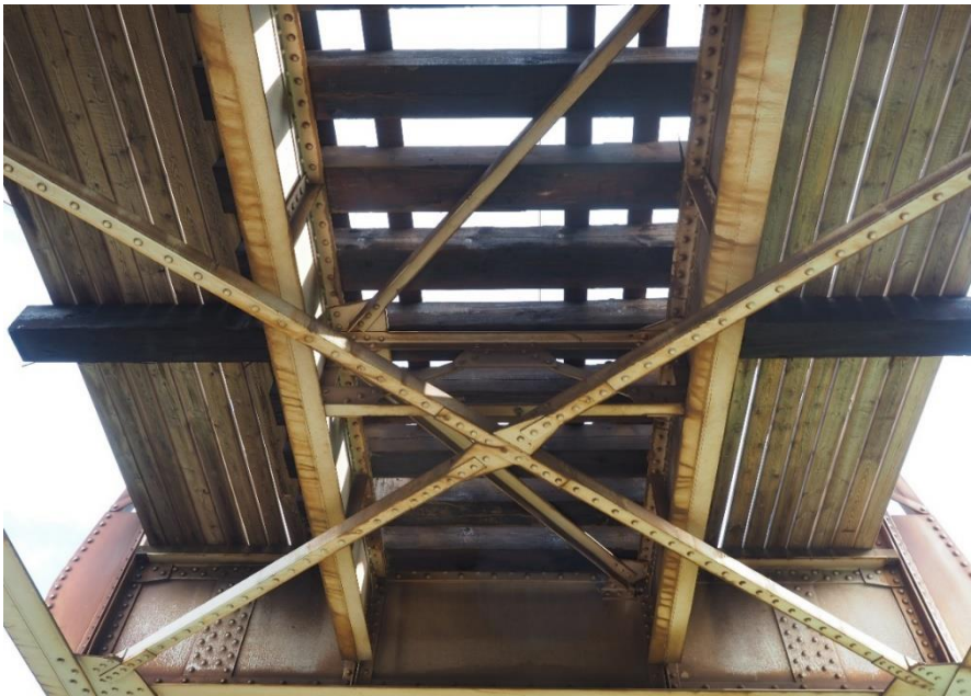
Figure 32, longer sleepers. Photo: Gunnstein Frøseth
