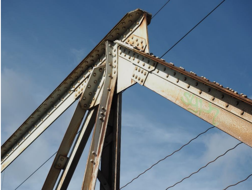
Figure 28, Top and end connection in truss. Photo: Gunnstein Frøseth
