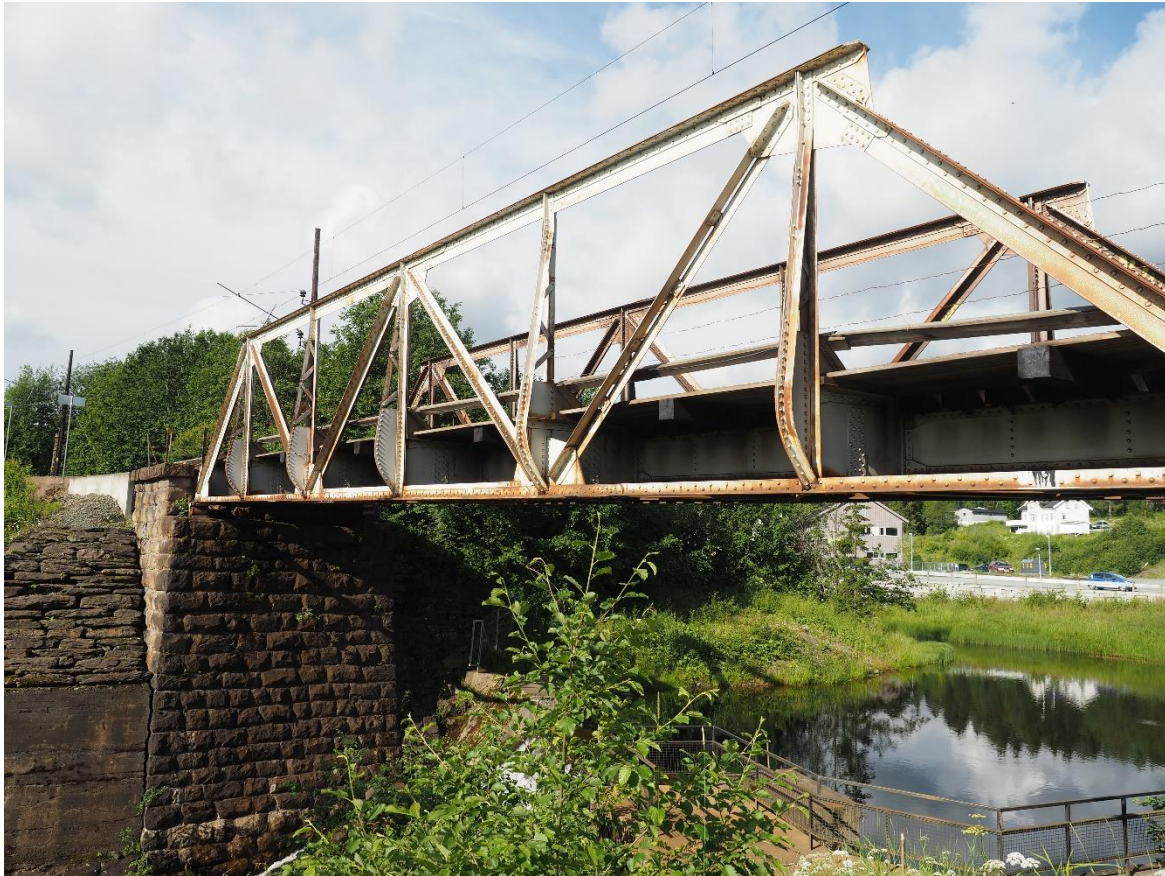
Figure 19, Lerelva Bridge. Photo: Gunnstein Frøseth
