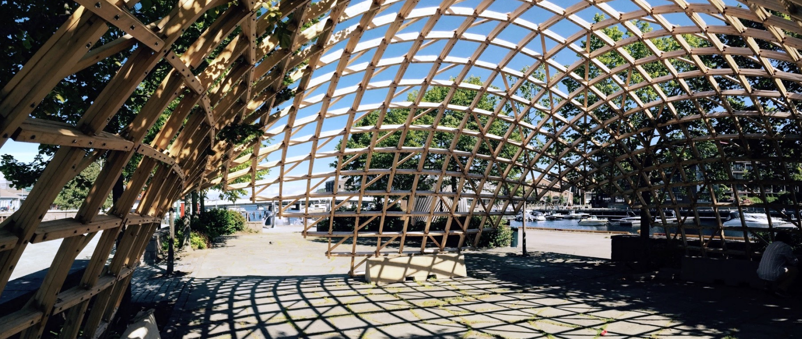
Figure 2.2: Grid shell by Steinar and John. Concrete blocks and the diagonal laths that were used to fix the structure is visible.
