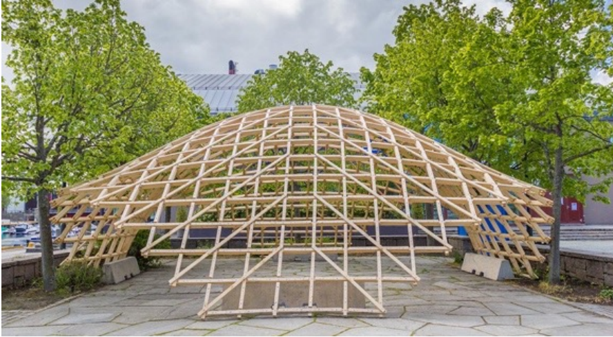
Photo 1 Photo of the gridshell pavilion built in Trondheim.
