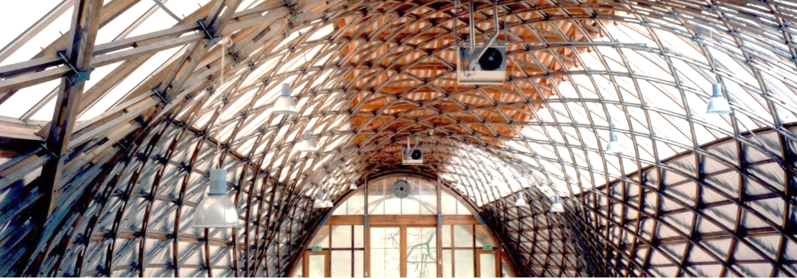
Figure 1.3: Downland Gridshell interior
