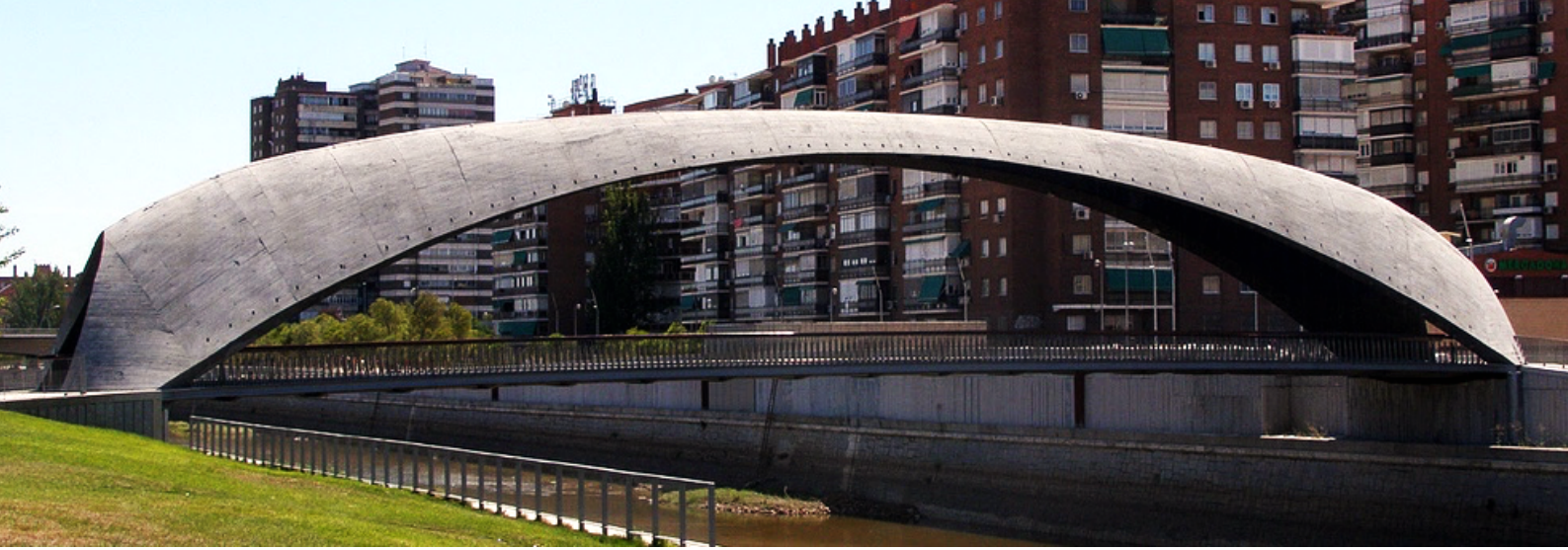
Figure 1.6: One of the shell bridges that span the Cascara river in Madrid.
