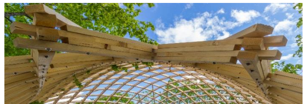
Figure 3: The original modular solution, detail from the experimental gridshell. Credits: Sophie Labonnote-Weber
