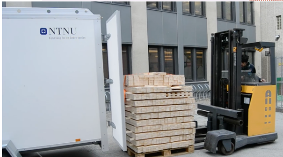
Photo 2 The segment lath makes transportation very compact. This image shows 50% of the modules in the built pavilion.
