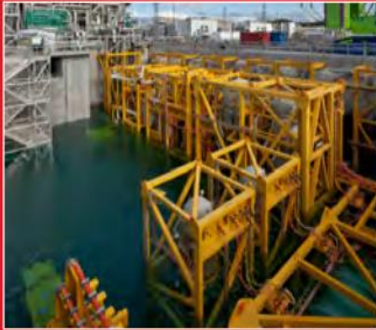
Fig. 1: Ormen Lange Pilot Compression Station
