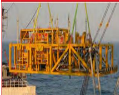
Fig. 6: Installation of the OneSubsea Multiphase Compressor Station for the Gulfaks Field
