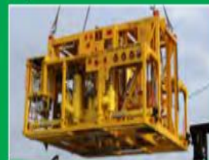
Fig. 9: Installation of the OneSubsea Pump Station for the Total Girri project
