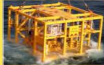
Fig.3: OneSubsea Raw Seawater Injection System being installed for Columbia E Field
