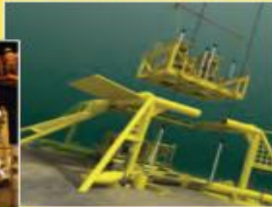
Fig. 2: Conceptual Illustration of Installation of Tyrihans Subsea Raw Seawater Injection (SRSWI) System
