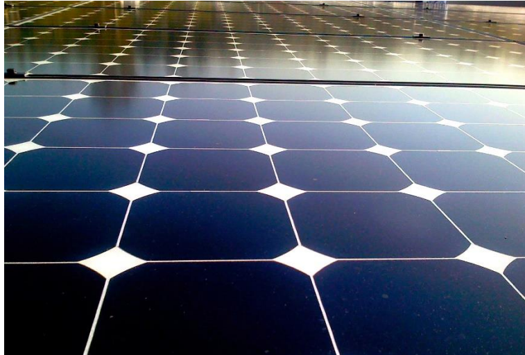
Figure 5. Interconnection of wafers in a solar module (11) .
