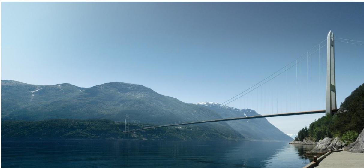
Figure 1.3: Complete picture of the entire bridge with pylons, cables and steel box girder [4].
