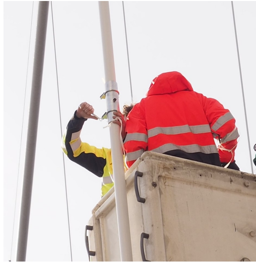
Figure 5.7: Installation of accelerometer on hanger 1
