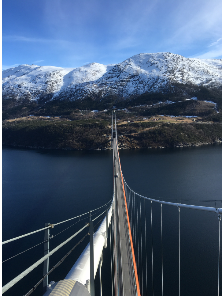
Figure 5.1: Day 1: Picture of bridge from tower.
