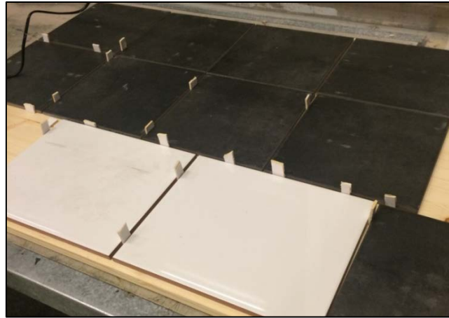
Figure 7-1: Tile layout strategy and spacing
