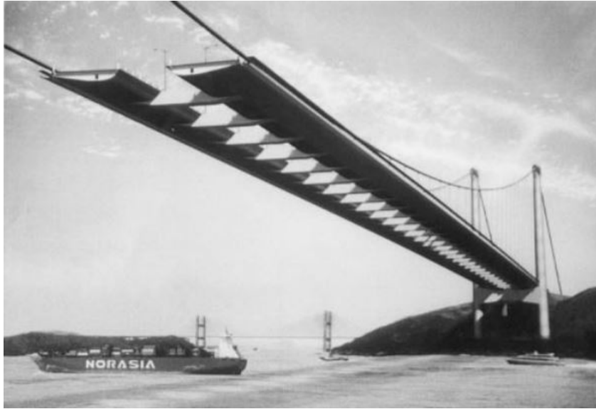
Figure 4.12: Conceptual design from 2002 of the Tsing Lung Bridge in Hong Kong [10]
