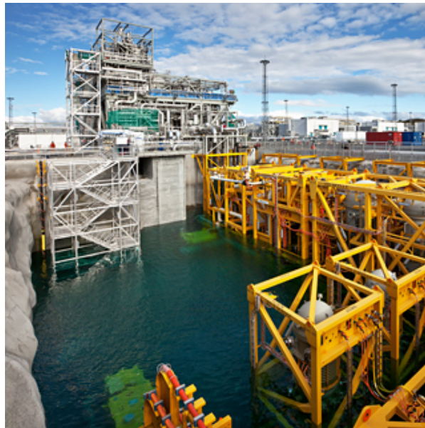
Figure 1.3: The Ormen Lange test pit [70].
