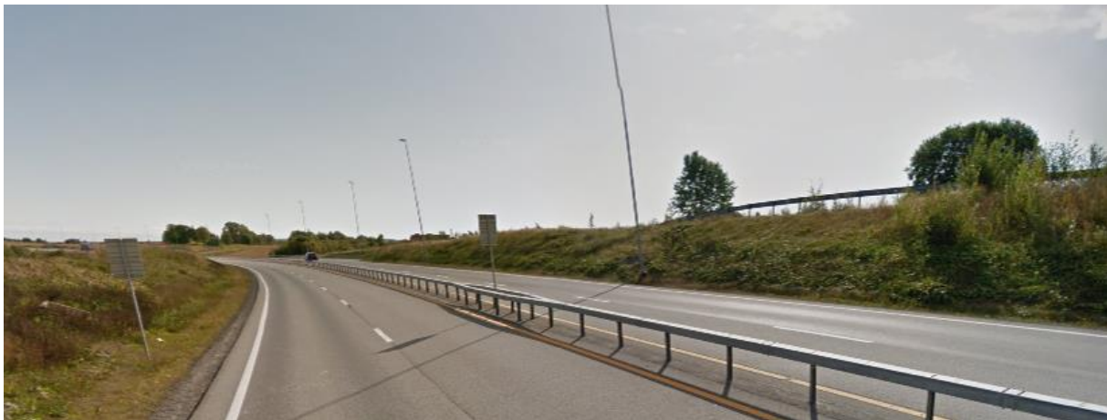
Figure 34: A picture of E16 between Kløfta and Nybakk. The picture is retrieved from ("google.maps [Picture]," 2016)
