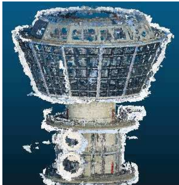
Figure 16 - Noises around the tower. They are concentrated on the metal shining parts.
