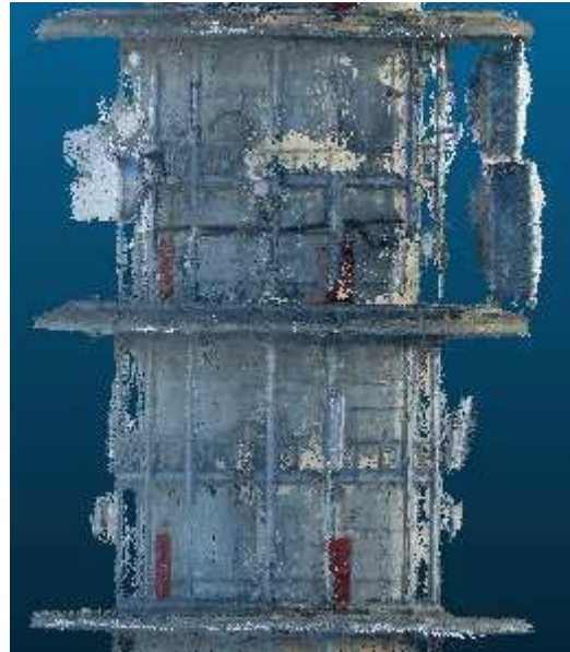
Figure 19 - Missing parts of the cylinder near support constructions.
