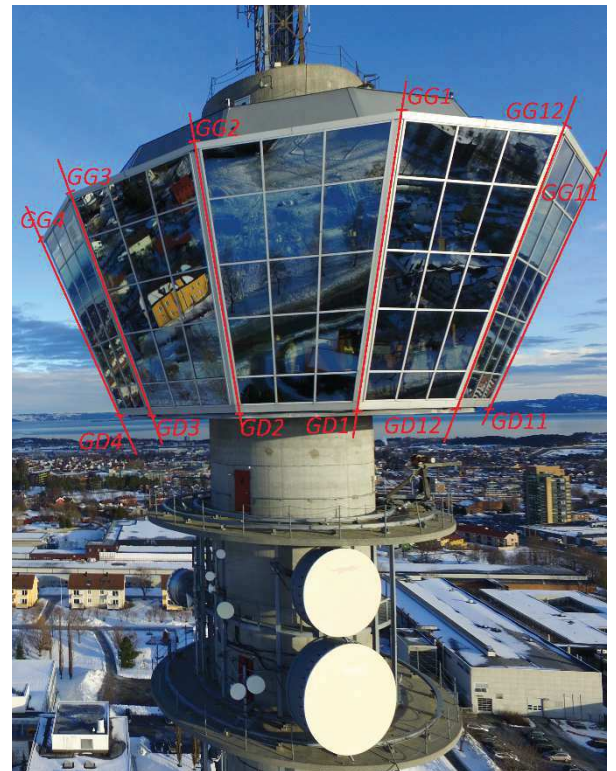
Figure 34 - Visualization of the scheme of a naming of GPCs. GG stands for the upper edge of the tower, GD for the bottom edge of the tower, and numbering of edges starts with the most south one and increasing clockwise.
