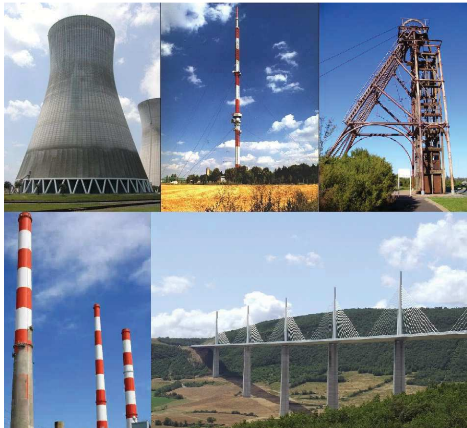
Figure 2 - Examples of high constructions [Multiple sources, google graphics.]
