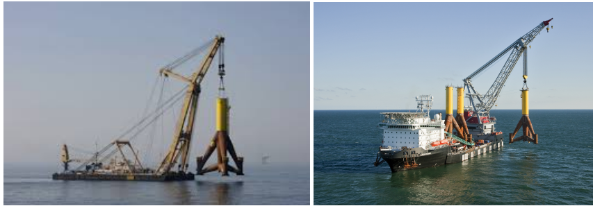
Figure 4.9: Lifting arrangement for tripod installation
