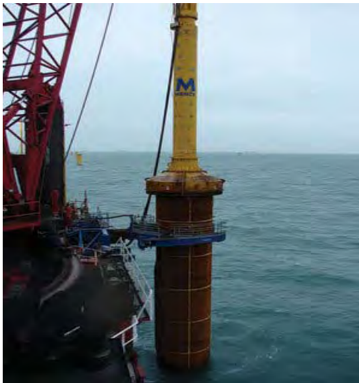
Figure 2: MP installation with gripper and Hammer on top.
