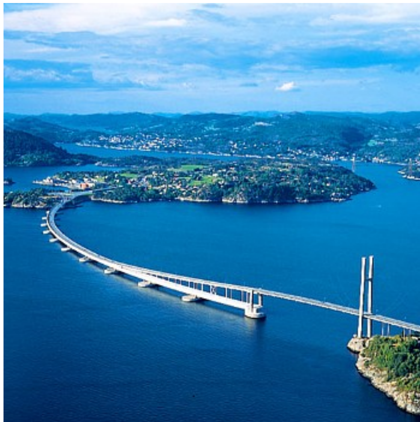
Figure 4: Nordhordaland bridge (NrK)
