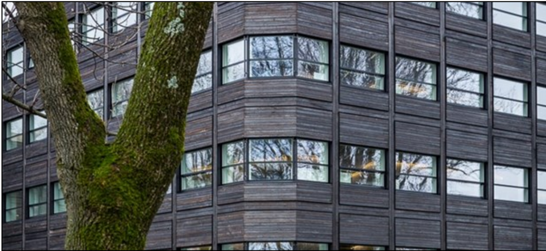
Figure 10.5: Exterior of Powerhouse Kjørbo
