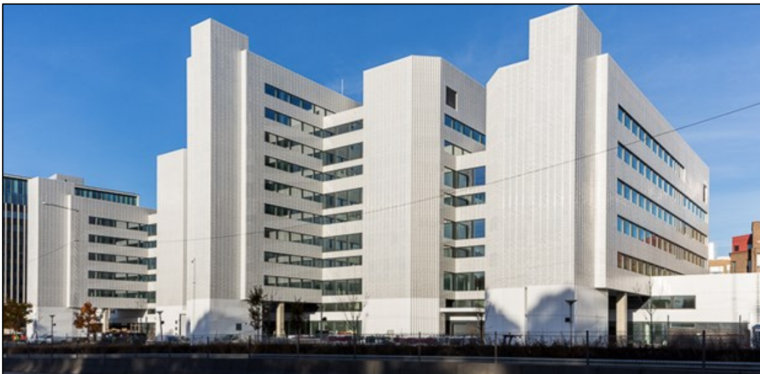
Figure 10.4: Exterior of Fredrik Selmers vei 4
