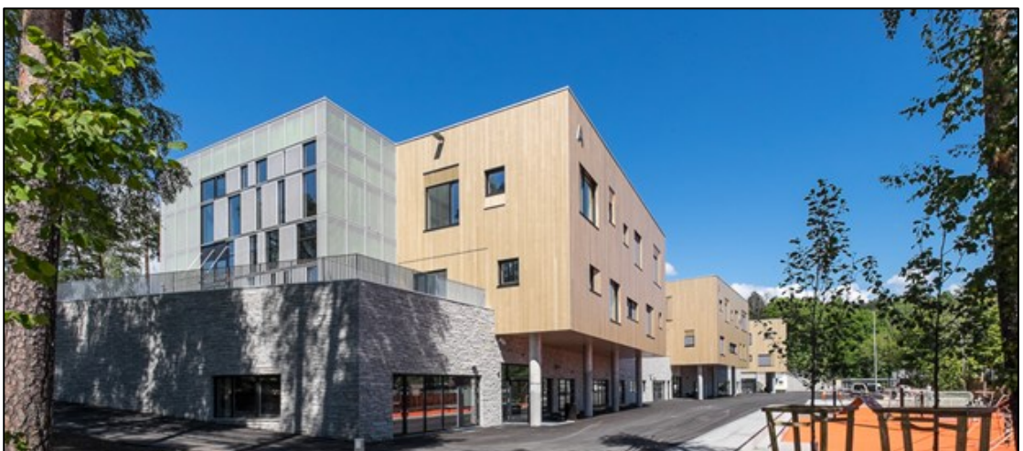
Figure 10.2: Exterior of Bjørnsletta School
